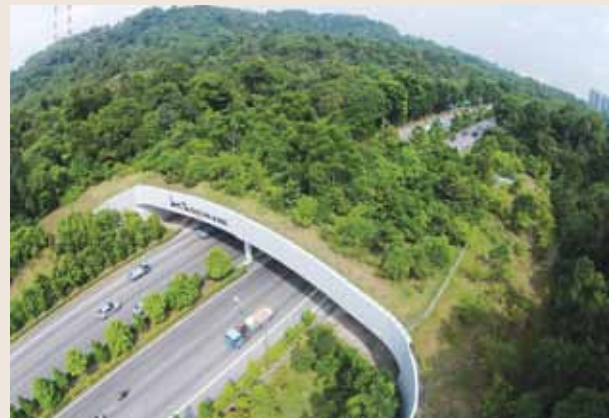
The Eco-Link@BKE in 2015, a bridge constructed in 2013 for wildlife to cross from the Bukit Timah Nature Reserve to the Central Catchment Nature Reserve
