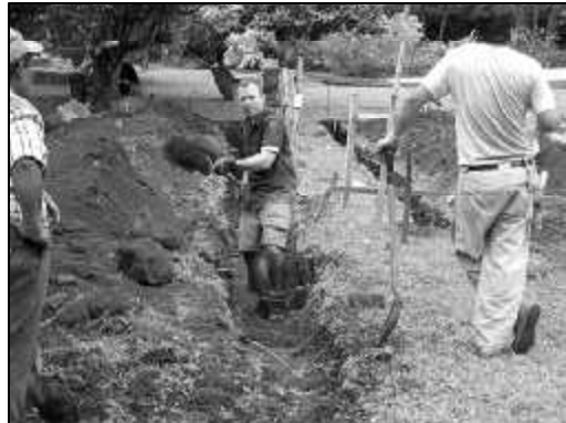
Breaking Ground at EVACC © Paul Crump
